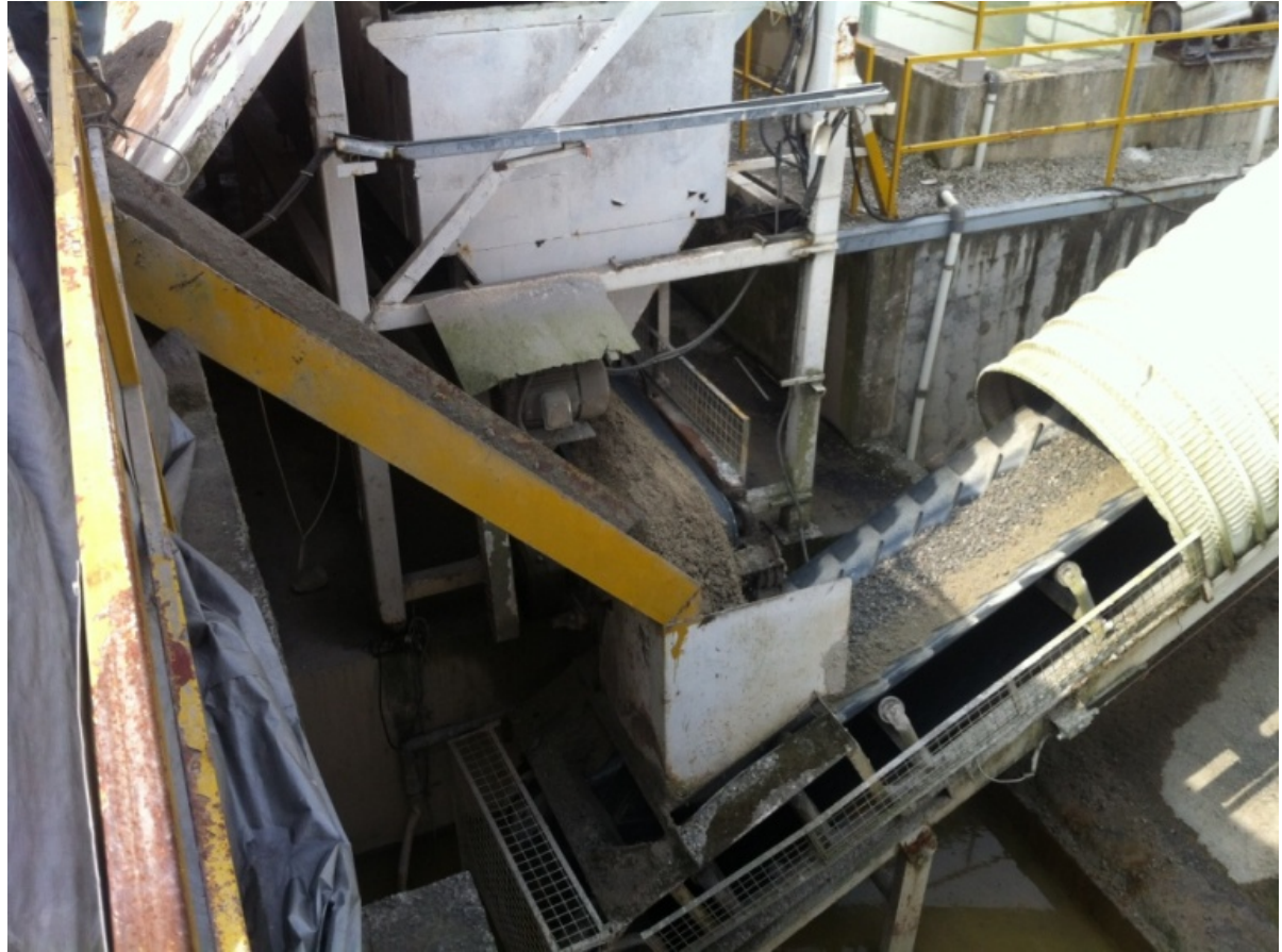
Adding ConMix into concrete mix at concrete plant.
